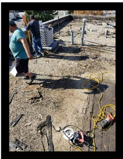
After removing 3 layers of old roofing they were able to fix the damages and lay the new roof down.
